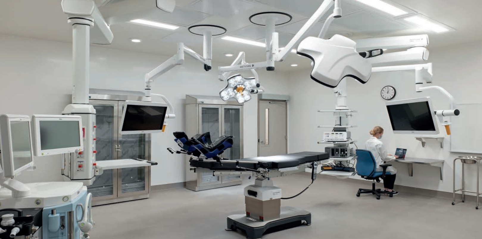
One of our satellite operating rooms (photo by Ben Rahn/A-Frame).
